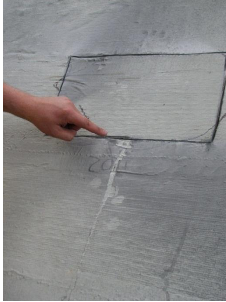
Figure 3.50. Water exiting the void area directly after the lower cut through the CFRP was completed
