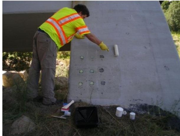
Figure 3.56. Applying a primer coat to the areas for repair
