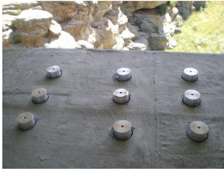
Figure 3.35. Adhered aluminum pucks for pull-off tests
