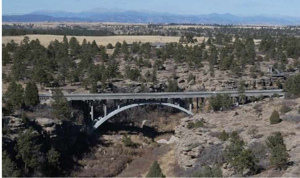
Figure 3.2. Castlewood Canyon Bridge (Mohseni, CDOT)
