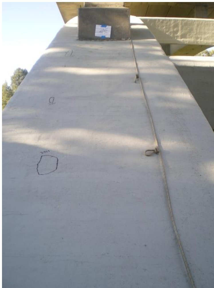
Figure A6. Bay 2NE, 3 Voids
