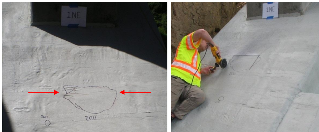
Figures 3.48 and 3.49. Void in CFRP with transverse crack identified with red arrows and Cutting the perimeter of the void in the CFRP
