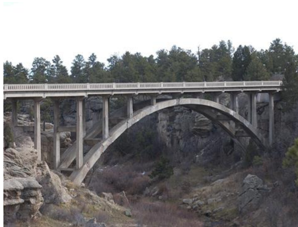
Figure 3.3. Castlewood Canyon Bridge prior to the 2003 repair (Mohseni, CDOT)
