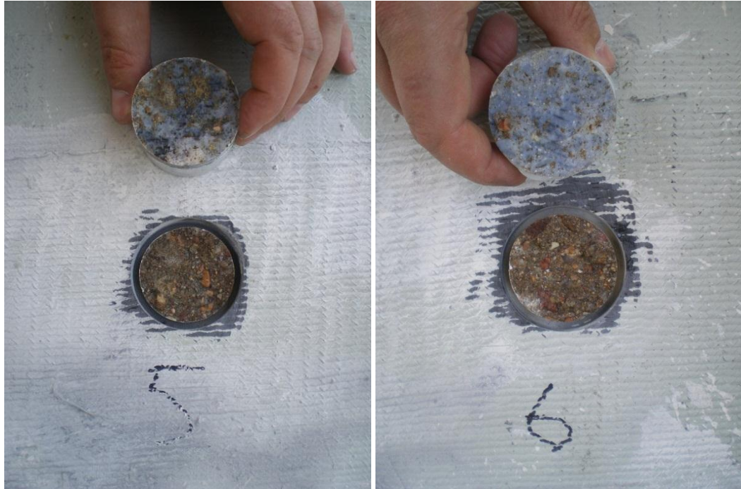
Figures B12 and B13. Test No.14, weak bond strength, and Test No.15, weak bond strength
