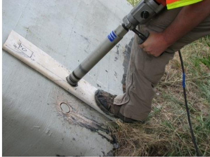
Figure 3.26. Starting a core hole using a wooden jig
