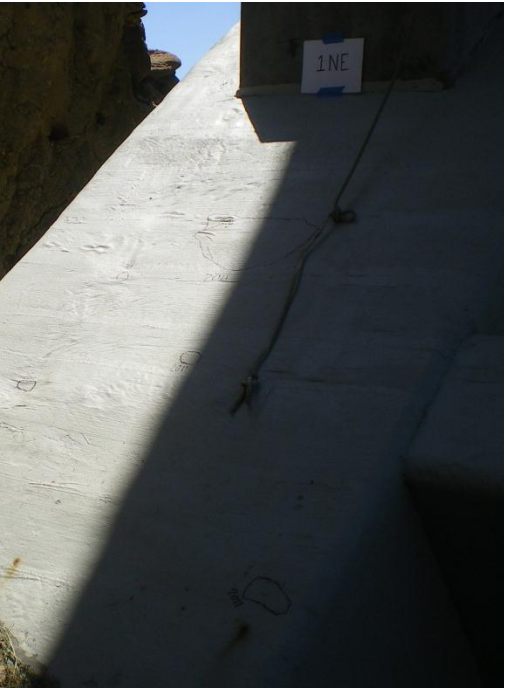
Figure A3. Bay 1NE, 5 voids
