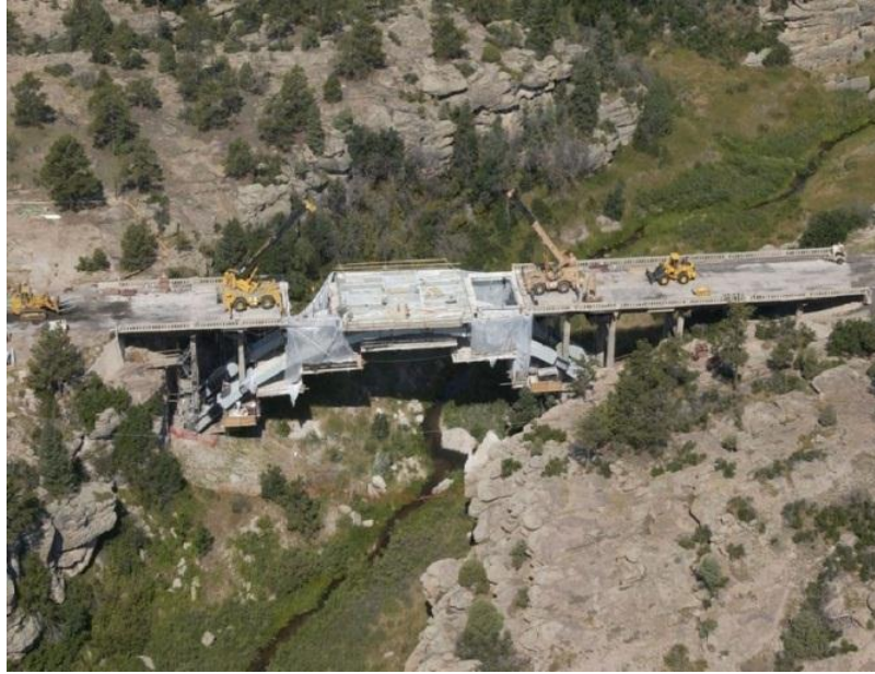
Figure 3.6. Systematically replacing the bridge deck (Mohseni, CDOT)
