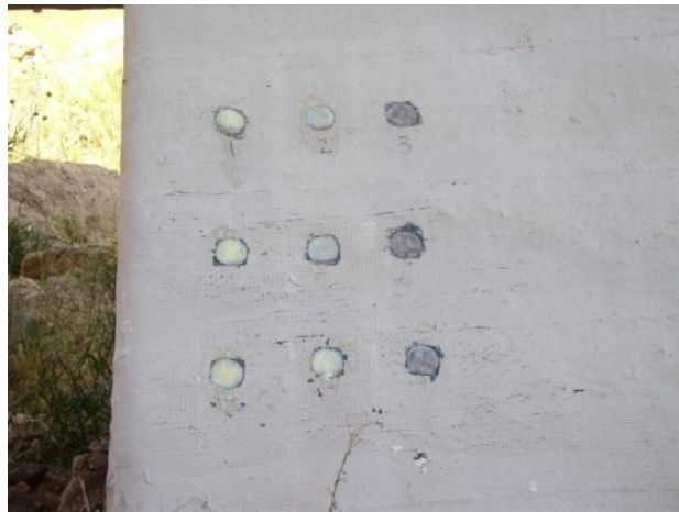
Figure 3.55. Epoxy filled holes following the pull-off tests
