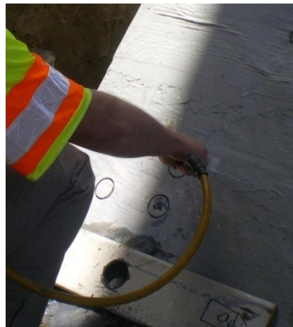
Figure 3.29. Removing water and debris from core cuts
